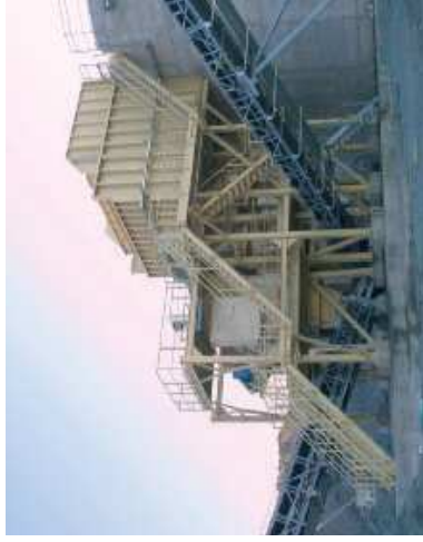
A C125 during the installation phase at a new primary crushing plant.
