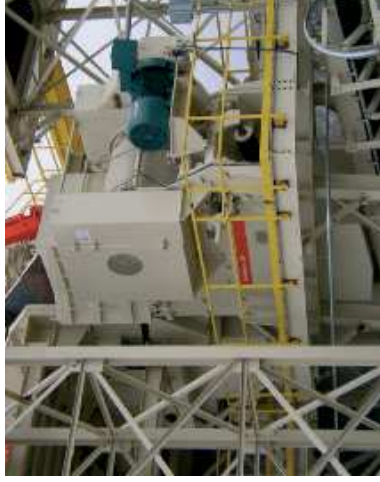
A C145 during the installation phase at a new primary crushing plant.
