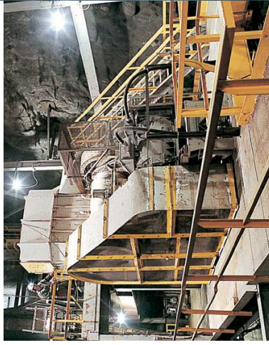
C160 at an underground gold mine.
