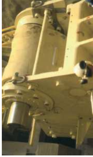
A Norberg C200 jaw crusher being assembled at an underground mine. The crusher was transported in pieces and assembled underground.
